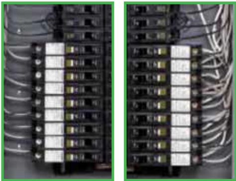
Plug-on Neutral Connections
