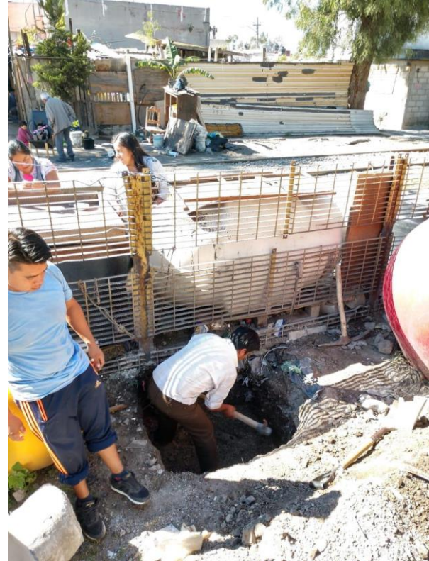
It takes several weeks and many neighbors to hand dig the footings. Precast footings are installed.
