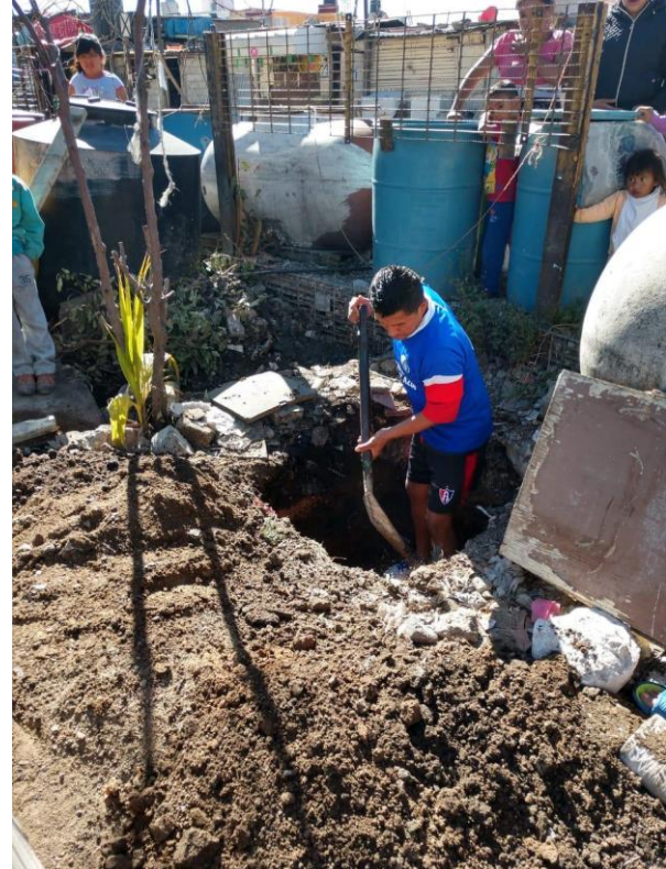
It takes several weeks and many neighbors to hand dig the footings. Precast footings are installed.
