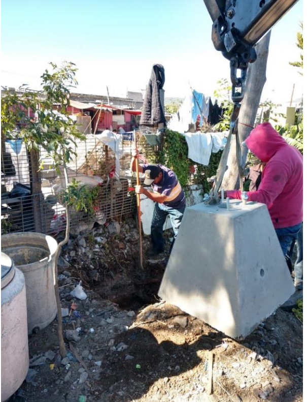
It takes several weeks and many neighbors to hand dig the footings. Precast footings are installed.
