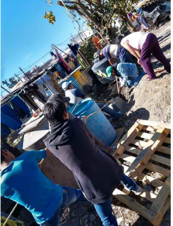
It takes several weeks and many neighbors to hand dig the footings. Precast footings are installed.
